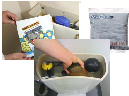
Reducing water in the toilet cistern
