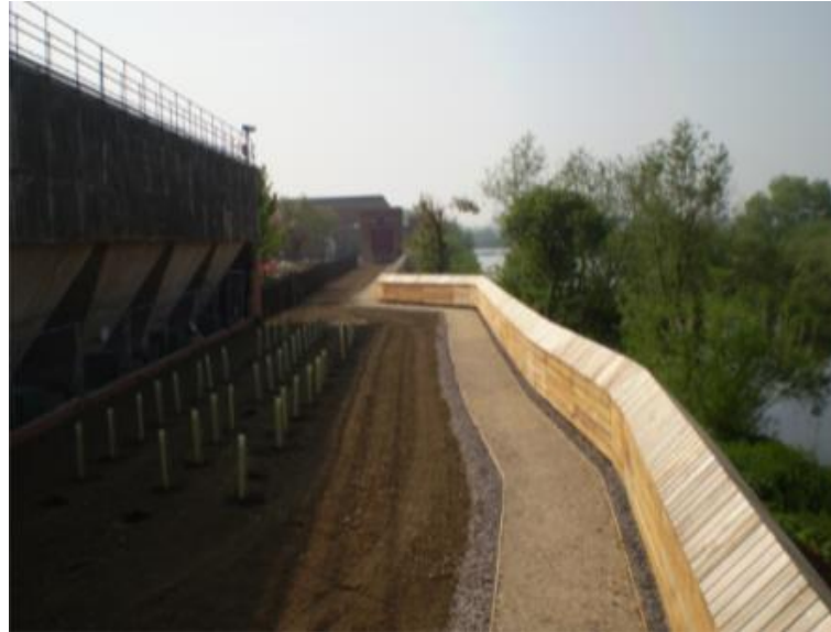
Flood defences constructed at Myth WTW
